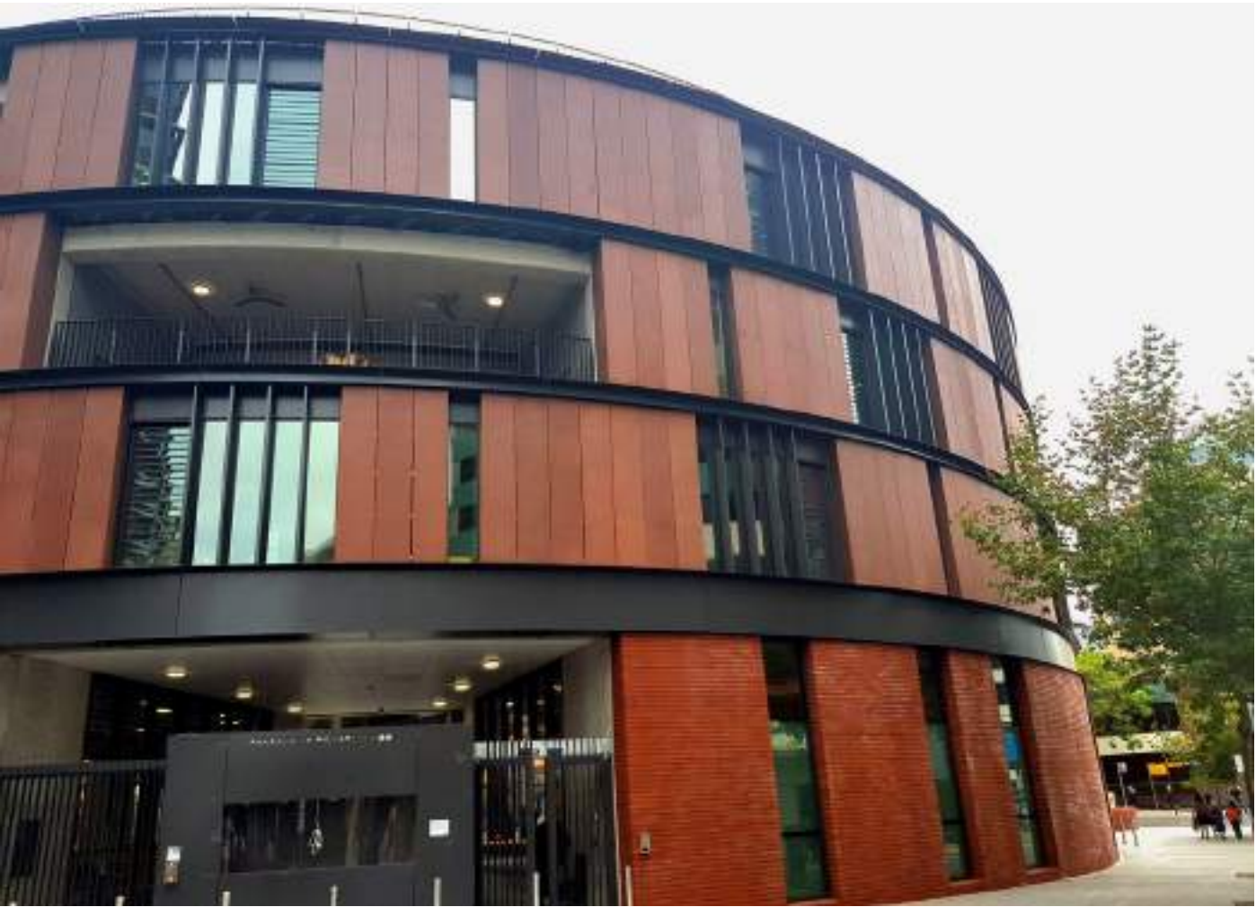
Parramatta Public School. Parramatta, NSW
